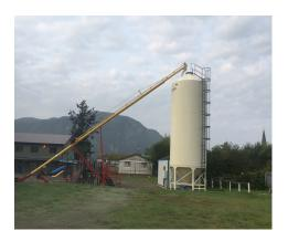
This is the new heating system for our school. There are 2 pellet-fed heaters in the powerhouse. The modified grain silo is to be filled with wood pellets that will feed it. The installation of the silo is yet to be completed.
